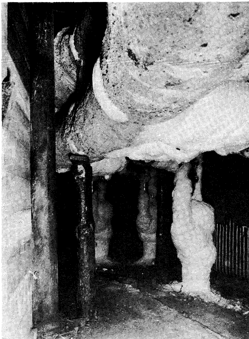
Photo A—Freeze chamber showing part of brine ring intake and return pipes (insulated) and some individual freeze pipes with ice formation.
